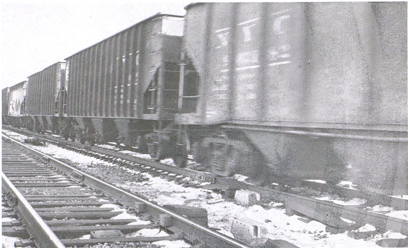
Double-direction detectors were initially installed on New York Central at Fairview, Pa., near Erie.
